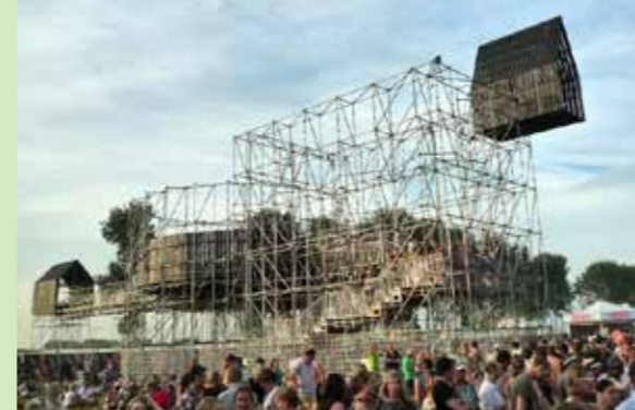
Scaffolding style system
